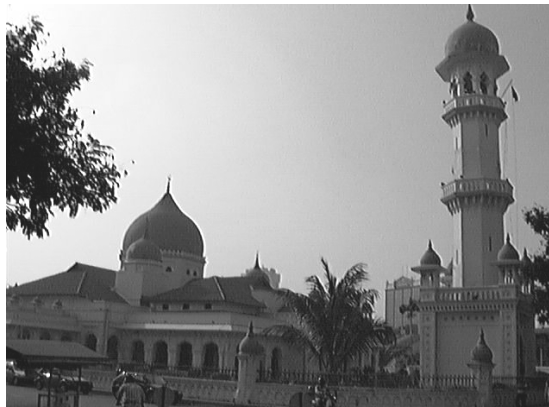
Figure 1 Kapitan Kling Mosque
